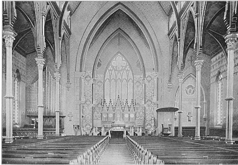
INTERIOR CHURCH OF THE ASCENSION—Northwest corner Massachusetts Avenue and Twelfth Street, N.W.
