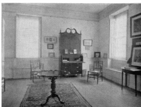
Plate LXIX.—Dining Room, Stenton; Library, Stenton.
