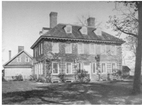
Plate IV.—Stenton, Germantown Avenue, Germantown. Erected by James Logan in 1727.
