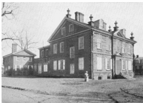
Plate XVII.—Cliveden, Germantown Avenue and Johnson Street, Germantown. Erected in 1781 by Benjamin Chew.
