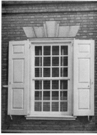
Plate XLIII.—Detail of Window and Shutters, Morris House.
