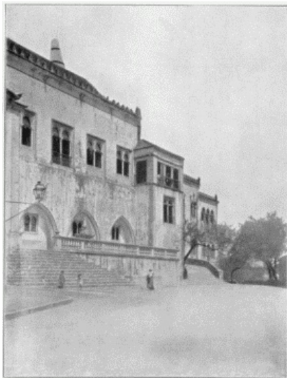
FIG. 44. PALACE, CINTRA. ENTRANCE COURT.
