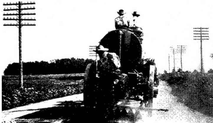
Fig. 20.—Oiling a Gravel Road
