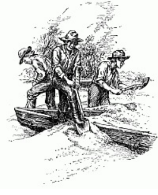
Digging out the scow.
