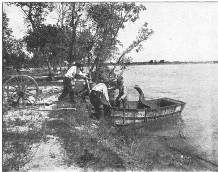
Launching the schooner to cross the river.
