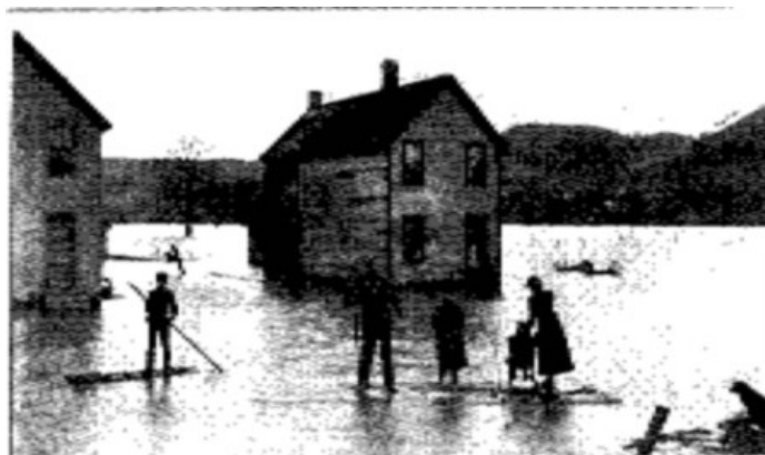
Fig. 2—Bad conditions about a dwelling.
