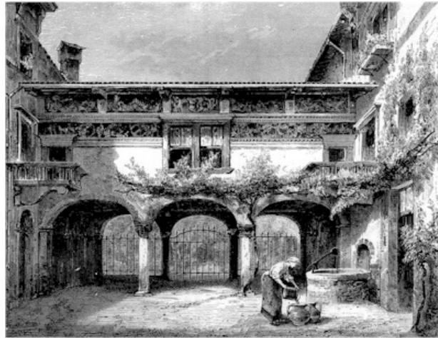
COURTYARD OF HOUSE IN VERONA
