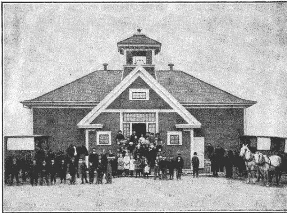
A frame building and adequate conveyances
