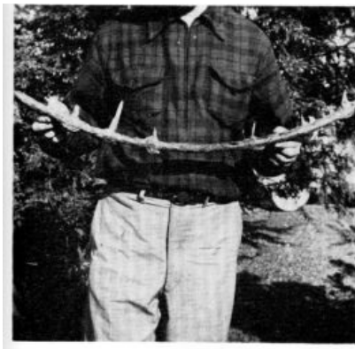
Figure 4.—A STRAKE, SHOWING SPIKES. On early vehicles the tires were put on in sections and spiked in place. Later one endless tire was "sweated" on by being heated to expand it, fitted on the wheel, and cooled in place.
