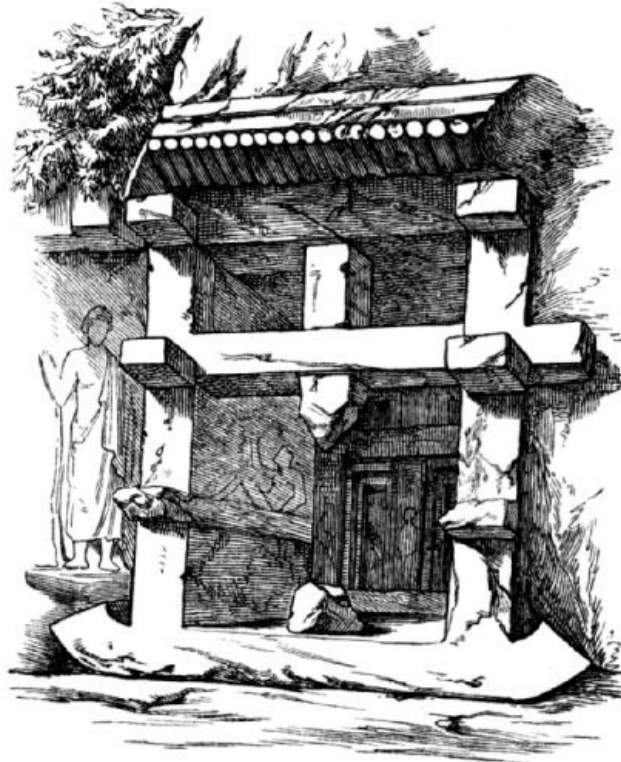
ROCK-CUT TOMB AT MYRA, IN LYCIA. Imitation of Timber Construction in Stone.
