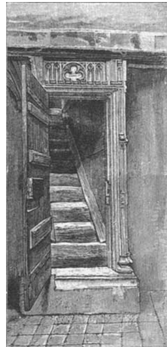
STAIRCASE TO WATCHING-GALLERY.
