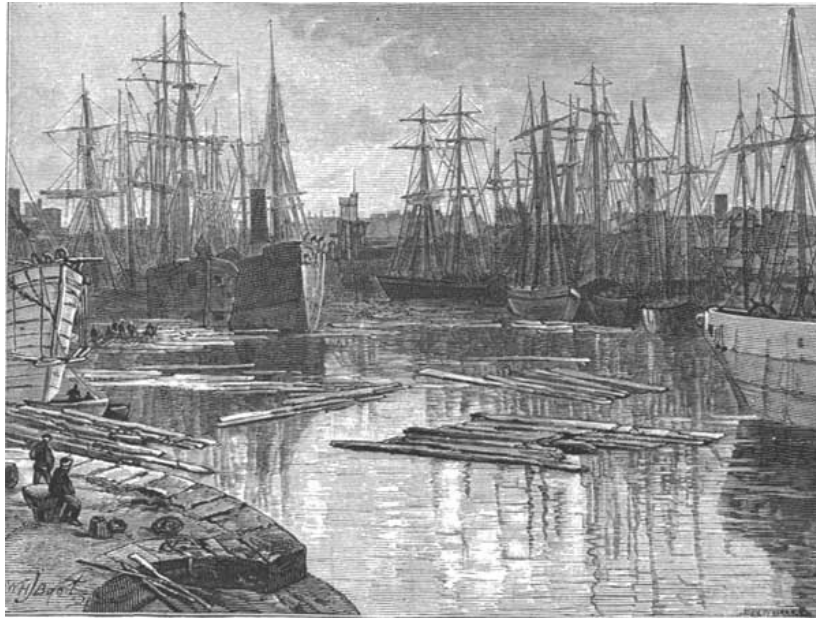
NORTH DOCK, SWANSEA.
