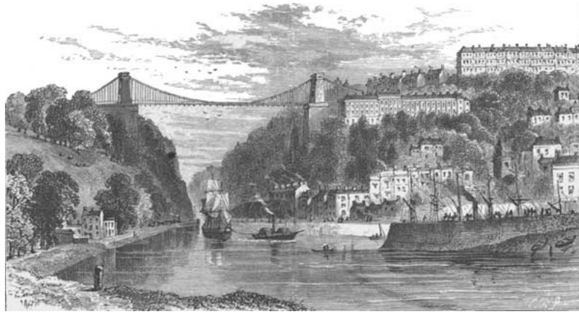
CLIFTON SUSPENSION-BRIDGE, BRISTOL.
