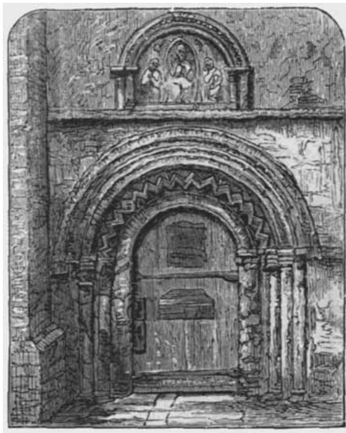
NORTH DOOR, ELSTOW CHURCH.
