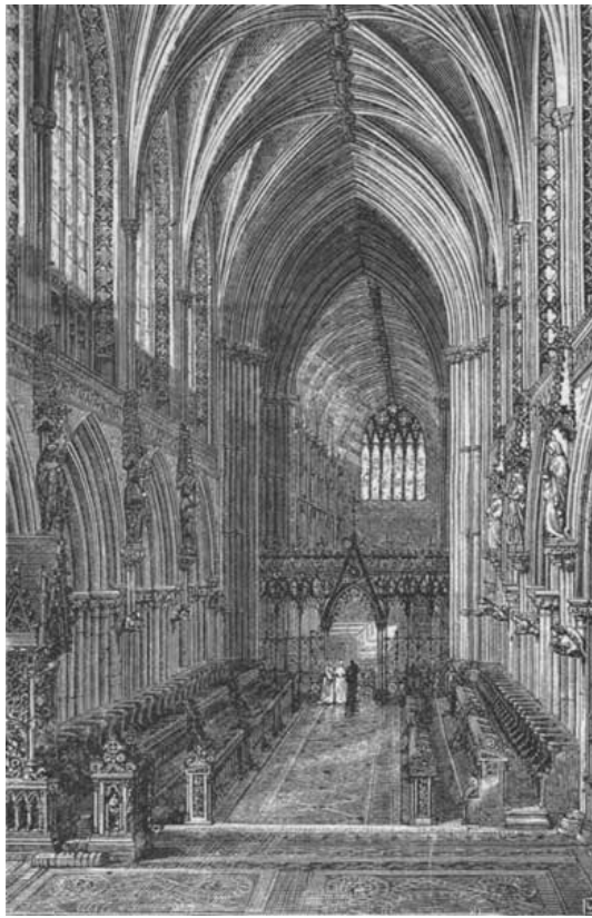
INTERIOR LICHFIELD CATHEDRAL, LOOKING WEST.
