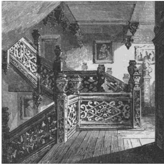
ELIZABETHAN STAIRCASE, HARDWICKE HALL.
