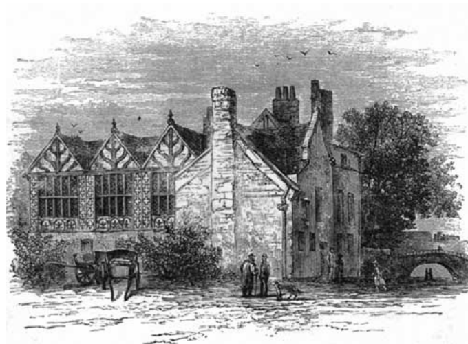
THE STANLEY HOUSE, REAR.
