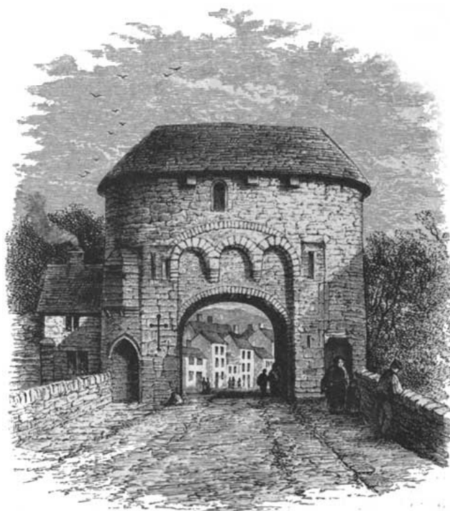
GATE ON MONMOUTH BRIDGE.
