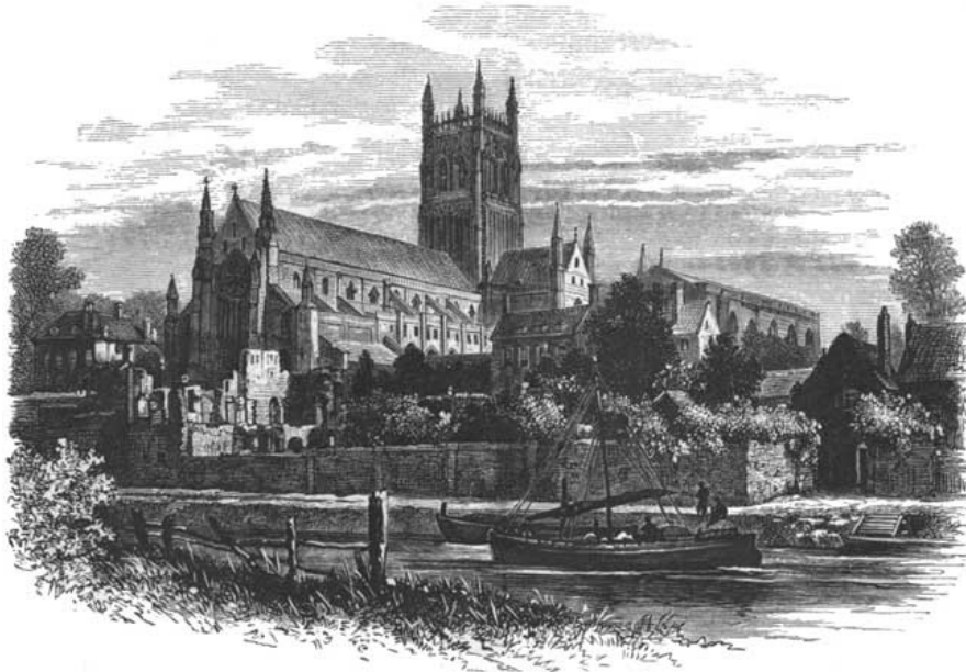
WORCESTER CATHEDRAL, FROM THE SEVERN.
