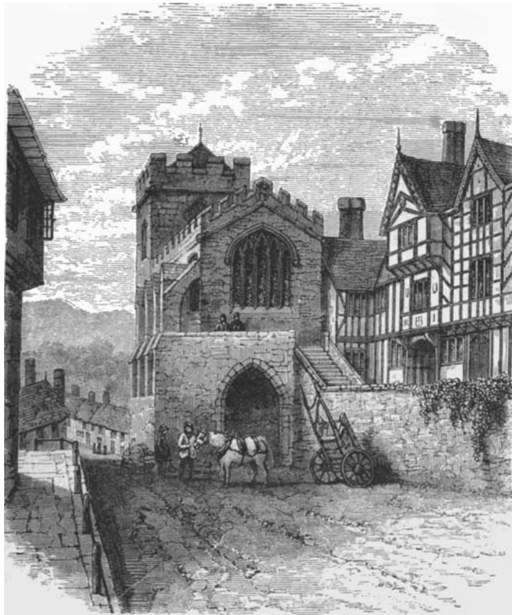
LEICESTER'S HOSPITAL, WARWICK.
