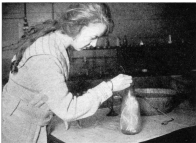
FIG. 166. The iron really burns in the jar of oxygen.
