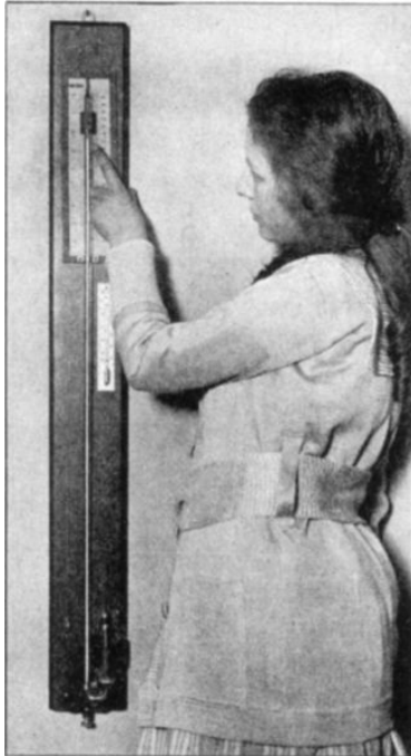
FIG. 155. The kind of mercury barometer that you buy.
