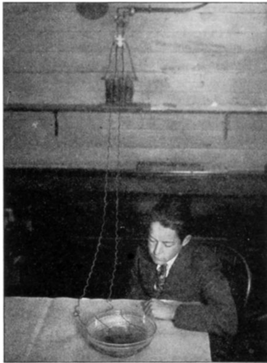
FIG. 178. Plating the copper by electricity.
