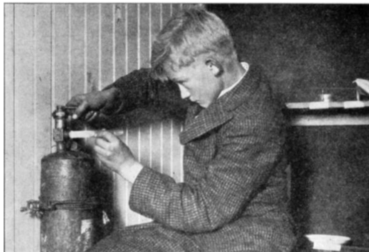
FIG. 46. The expansion of the compressed gas freezes the moisture on the tube.
