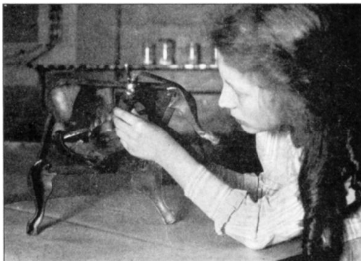
FIG. 169. Regulating the air opening in a gas stove.
