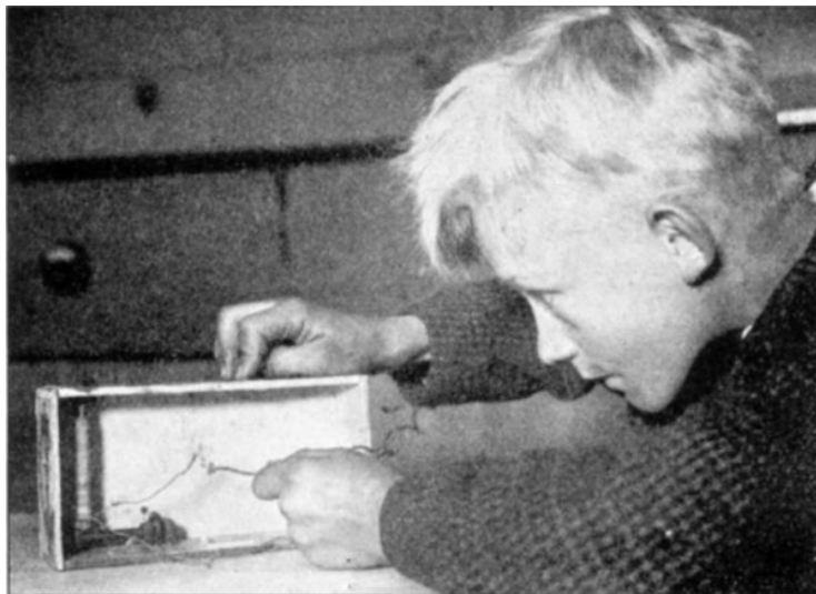
FIG. 139. Sending a message with a cigar-box telegraph.
