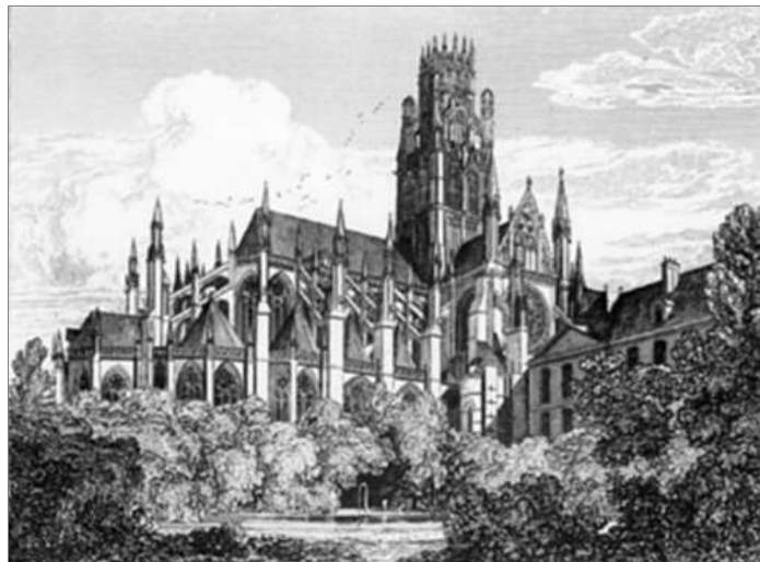
Plate 76. ABBEY CHURCH OF ST. OUEN, AT ROUEN. North East View.
