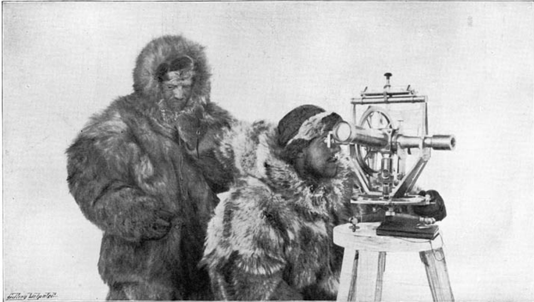
A chronometer observation with the theodolite
