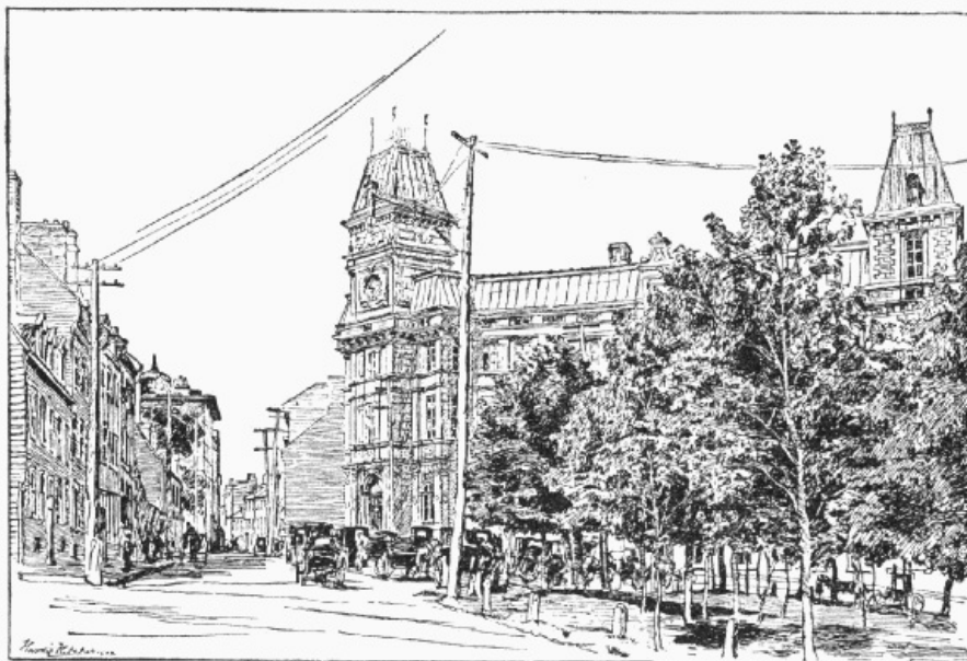
ST. LOUIS STREET, PLACE D'ARMES, AND NEW COURT HOUSE
