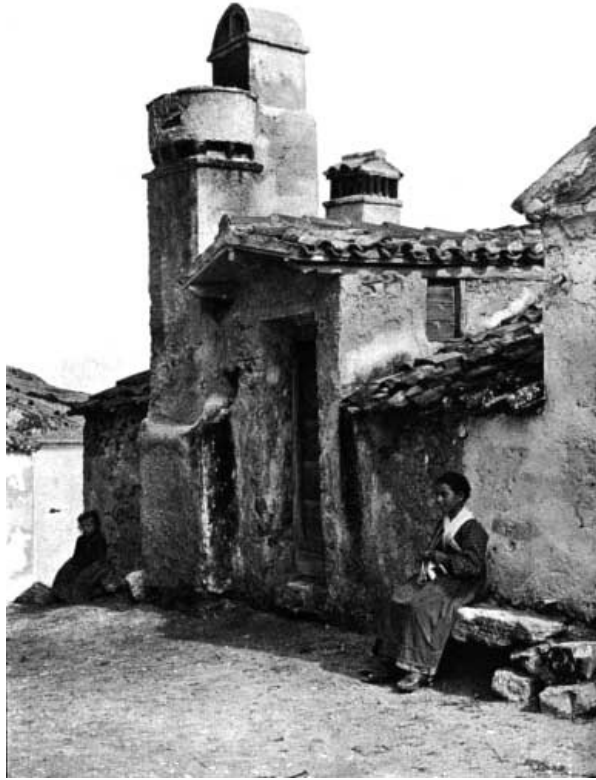
CHIMNEYS AT BESCA NOVA
