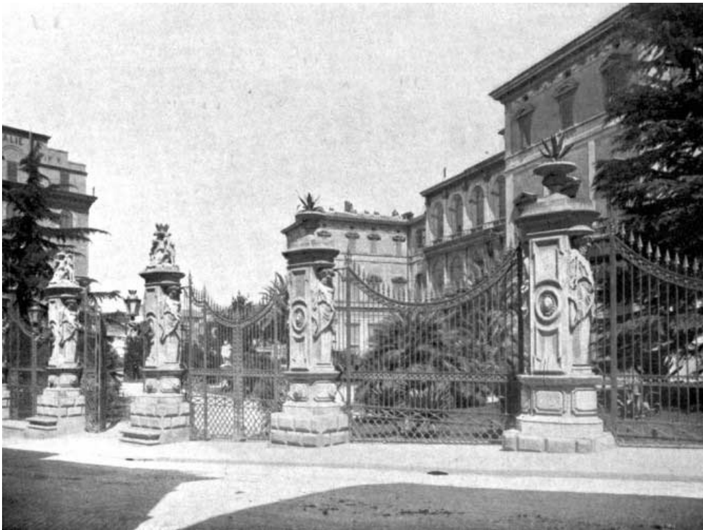
THE PALAZZO BARBERINI, VIA QUATTRO FONTANE, ROME. The home of William Wetmore Story and his family for nearly forty years.
