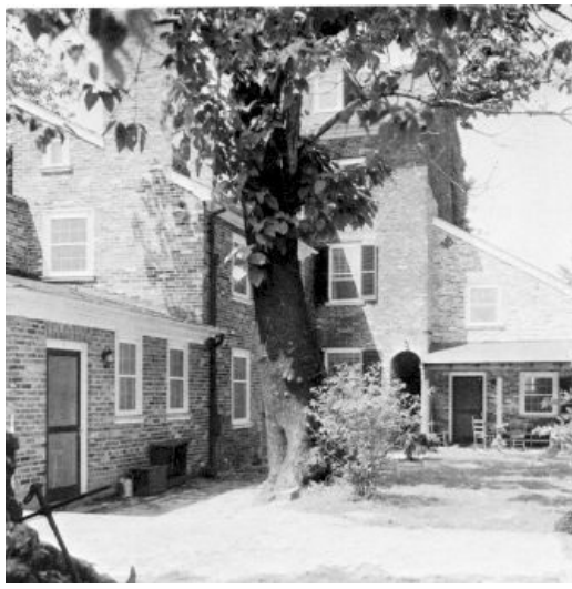
Rear of house and courtyard built by John B. Murray and bought by Dr. James Craik. The leanto at right replaces the frame building of Joseph Robinson, sailmaker
