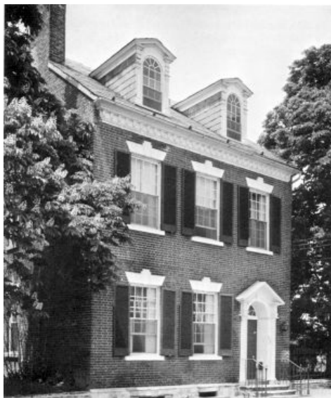
The Vowell-Snowden House. The widow's walk is missing
