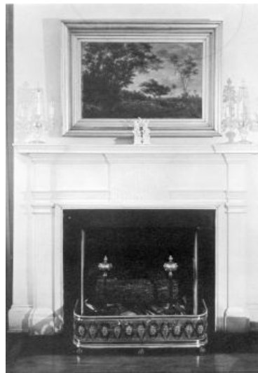
Mantel in the home of the late Mr. and Mrs. Norman H. Davis, 804 Prince Street. Late 18th and early 19th Century reeded carving, typical of the Federal House. The decoration is achieved by the returns around the pilasters, the reeded trim and diamond motif in the center panel.
