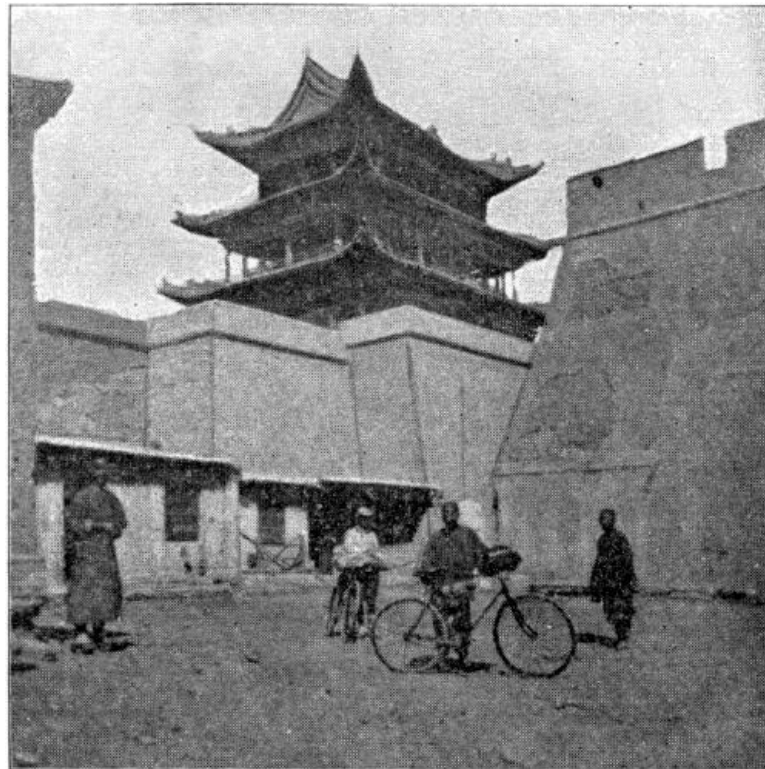
WITHIN THE WESTERN GATE OF THE GREAT WALL.
