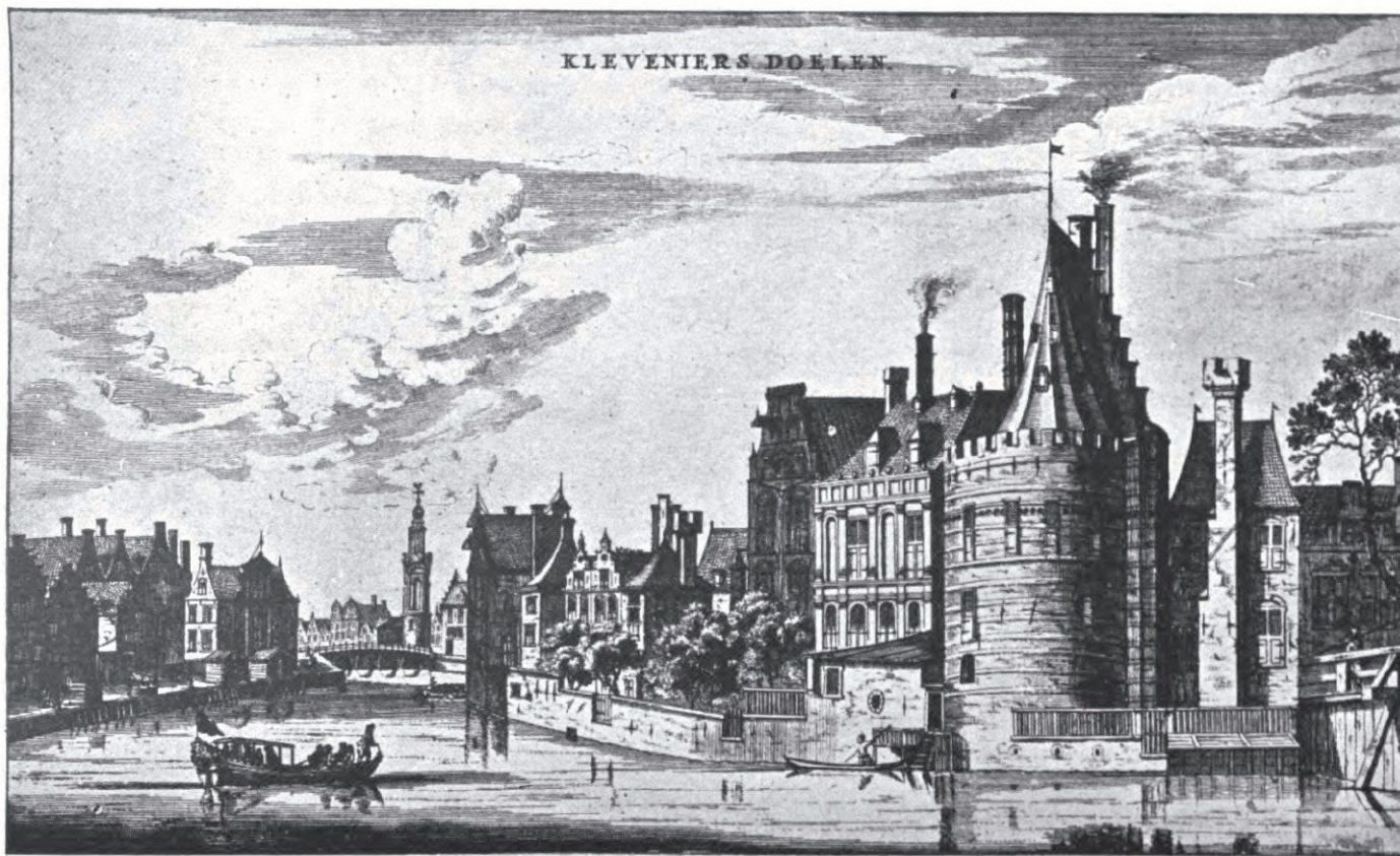
Plate 20. The Tower "Swyght-Utrecht" and the Backs of the Houses of the "Doelenstraat" in Amsterdam. The third house from the tower must be the one occupied by Rembrandt in 1636. After an engraving by van Meurs of about 1660.
