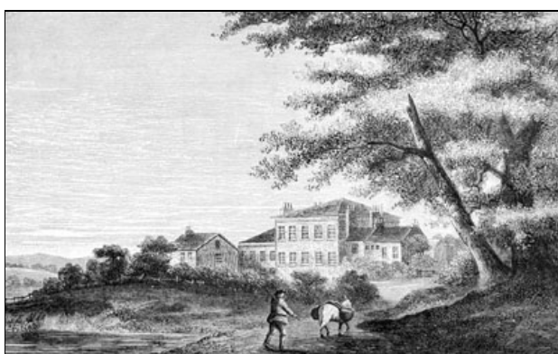
ORIGINAL BUILDING OF THE RETREAT, YORK. INSTITUTED 1792.
