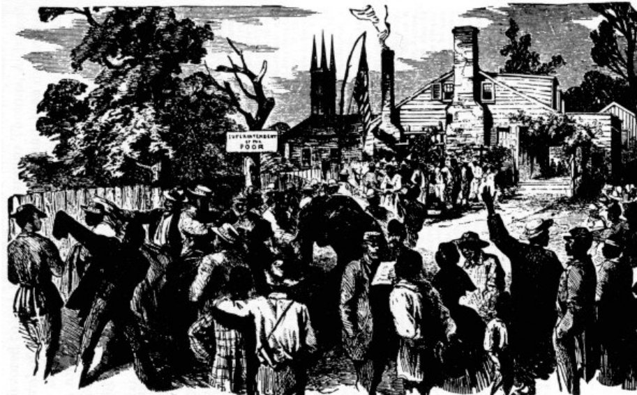
HEADQUARTERS OF VINCENT COLLYER, SUPT. OF THE POOR AT NEWBERNE N. C. Distributing clothing, captured from the Confederates, to the free negroes.
