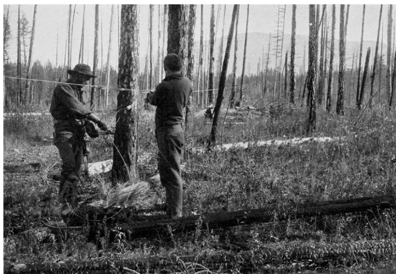
STRINGING A FOREST TELEPHONE LINE
