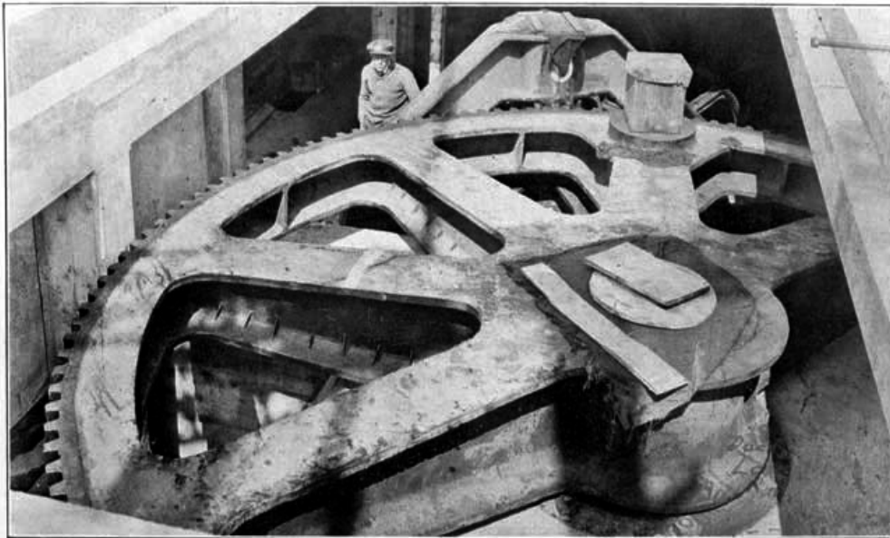
BULL WHEEL Part of Operating Machinery for Lock Gates
