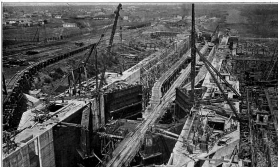
BUILDING THE LOCK
