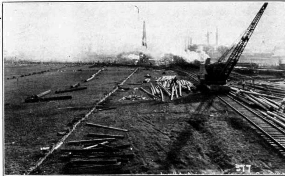
LOCK SITE Driving Sheet Piling
