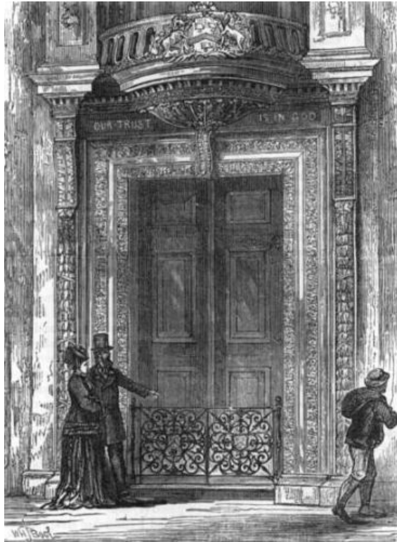
THE DOOR OF SADDLER'S HALL
