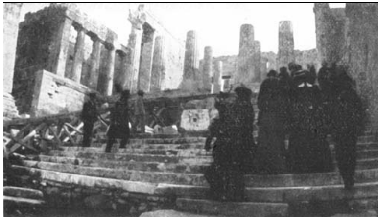
ONCE THE MAGNIFICENT MARBLE STAIRCASE.
