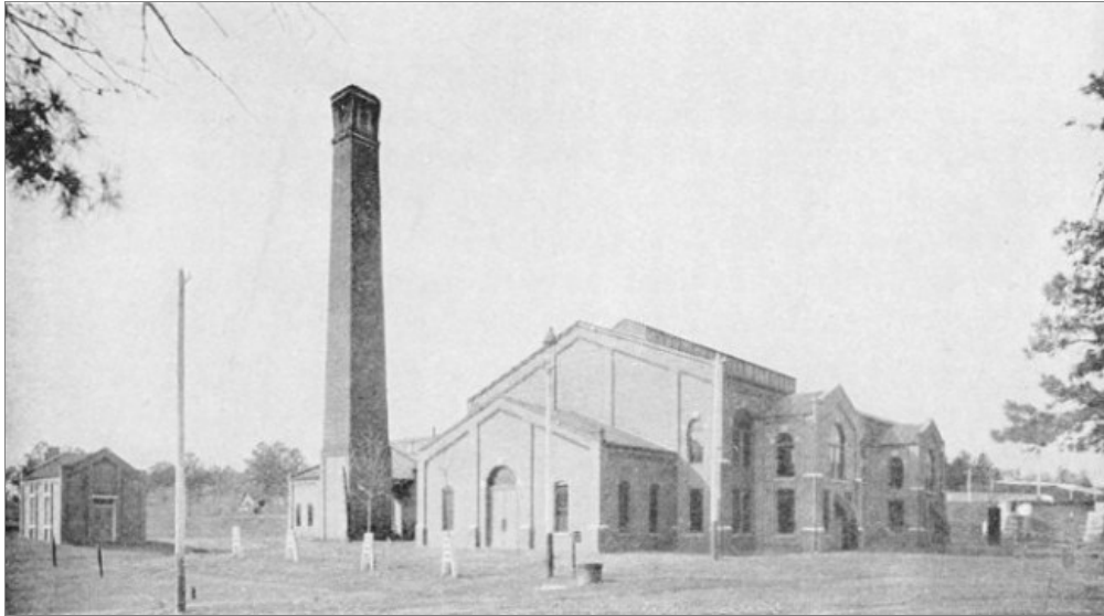
WATER WORKS PUMPING STATION.
