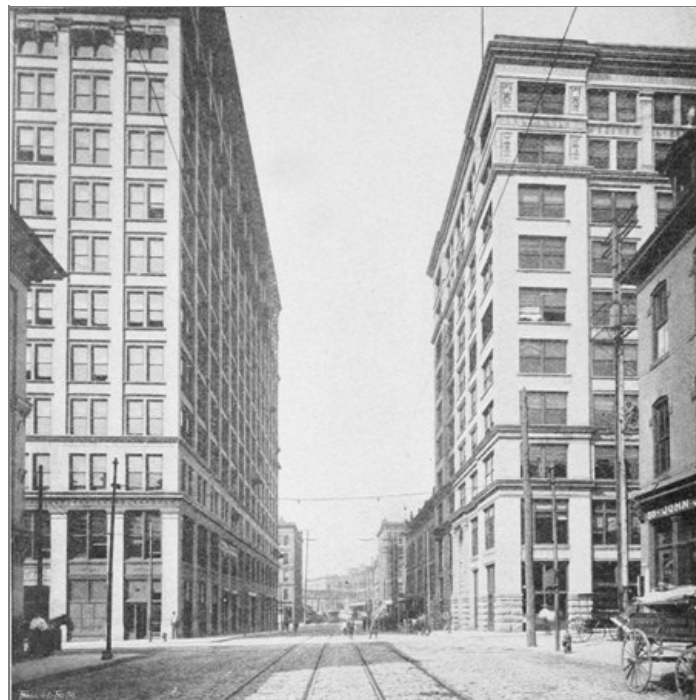
PRUDENTIAL AND EMPIRE BUILDINGS.
