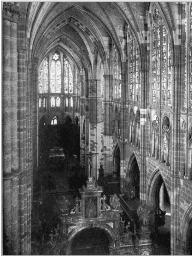
CATHEDRAL OF LEON Looking up the nave
