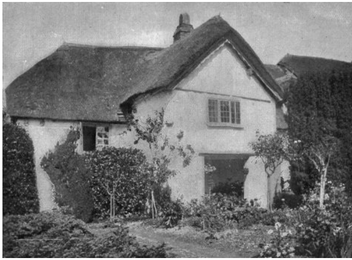
COB HOUSE TEMP. ELIZABETH, LEWISHILL. Walls from 3 ft. to 4 ft. thick. A wing was added in 1618. This farm has been occupied by the family of the present holder between 300 and 400 years.
