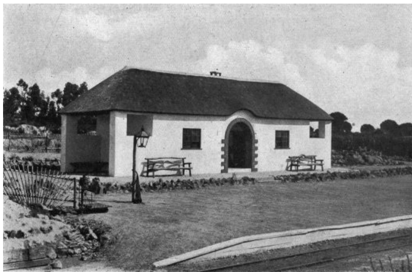
WAYSIDE STATION OF PISÉ AT SIMONDIUM, SOUTH AFRICA, DESIGNED BY MR. HERBERT BAKER.
