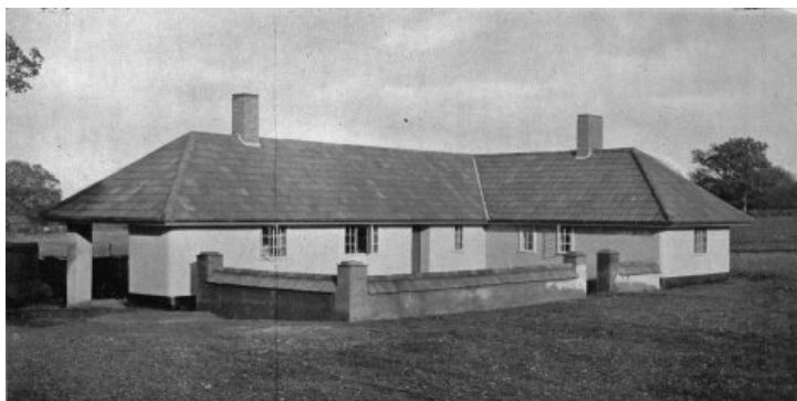
THE NEWLANDS CORNER PISÉ DEMONSTRATION BUILDING.
