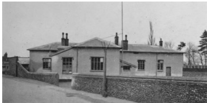
ONCE CORN HALL, NOW COUNCIL SCHOOL. Built about a hundred years ago. Still in sound condition and quite dry.
