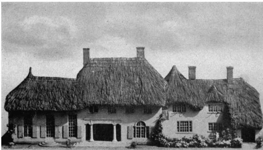
MODEL OF A PISÉ DE TERRE HOUSE TO BE BUILT IN THREE SUCCESSIVE STAGES. The right wing is planned to be built first as a complete small cottage, eventually becoming service and servants' quarters.
