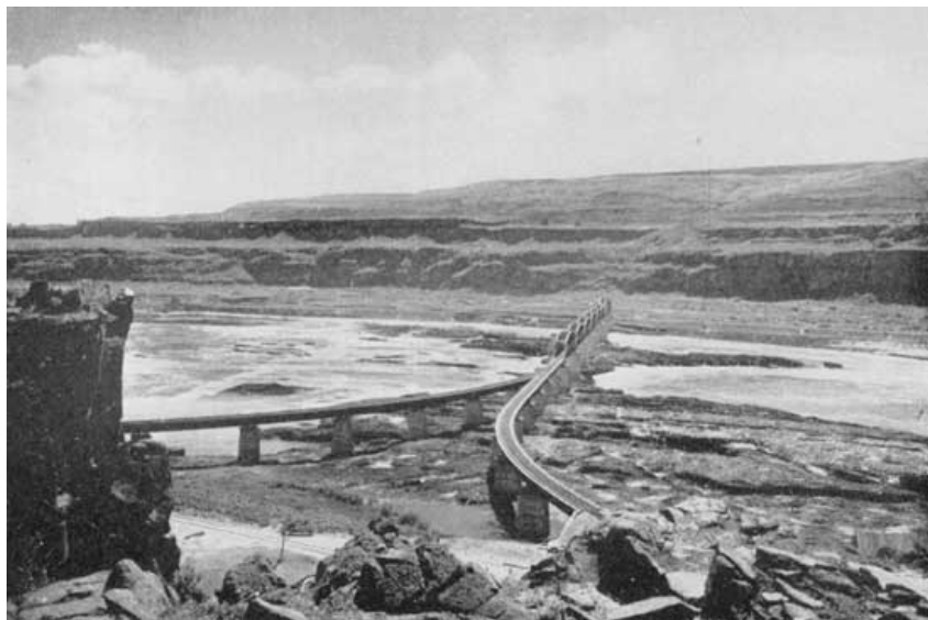
Where the Oregon Trunk Railway crosses the Columbia. "The river rolls between banks of barrenness"
