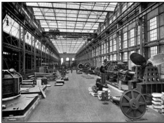
HARLAND AND WOLFF'S TURBINE ERECTING SHOP
