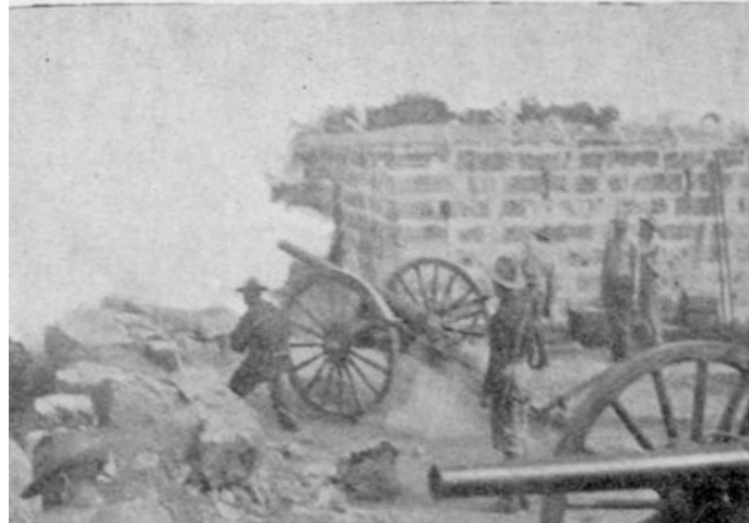
GUN AT PUMPING STATION FIRING ON MARIQUINA.
