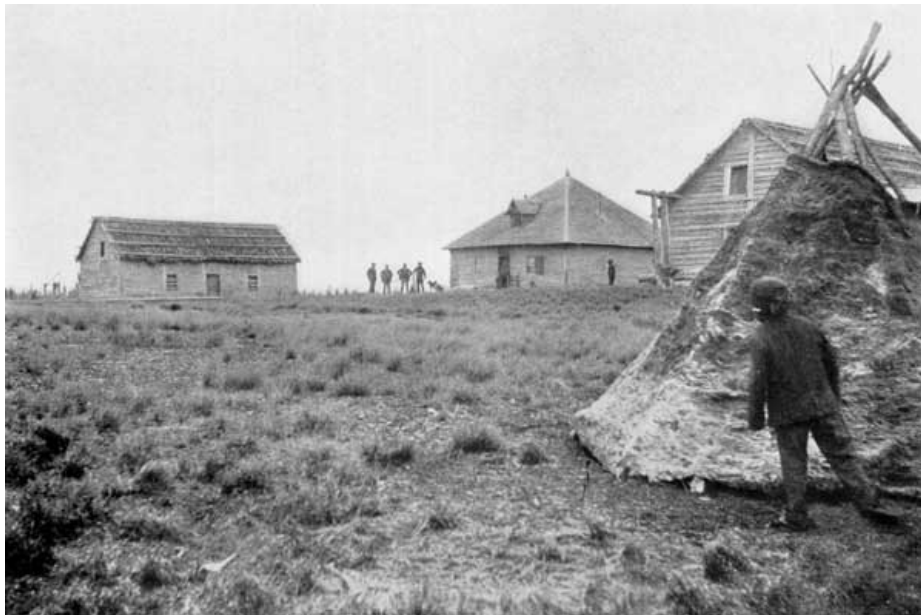
Fort MacPherson, now the most northerly post of the Hudson's Bay Company, beyond tree line; hence the houses are built of imported timber, with thatch roofs.
