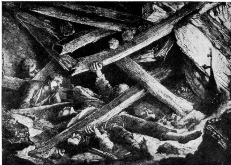
FALLING-IN OF A MINE.
