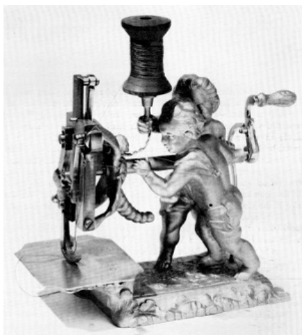
Figure 42.—THE FOLIAGE SEWING MACHINE originated with D. W. Clark. Once again he did not include the design in his June 8, 1858, patent, which was aimed at improving the feeding
