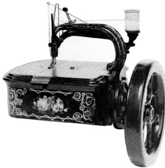
Figure 33.—SINGER FAMILY MACHINE, 1858, head only. (Smithsonian photo 45524-F.)
