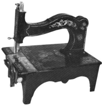
Figure 81.—EUREKA SEWING MACHINE, 1859. An example of the many short-lived types of which no written record can be found, this particular machine was used as a patent model for certain minor improvements in 1859. It has the name "Eureka" painted on the top and the following inscription incised on the baster plate: "Eureka Shuttle S. M. Co. 469 Broadway, N.Y." Although it is a shuttle machine, it carries no patent dates and was not included in the Howe royalty records. Neither is it listed in the obsolescence list published in 1881. The company probably could not pay its royalty fees and was forced out of business almost immediately. If this machine had not been used as a patent model, no record of the company's existence might remain. It should be noted that as in most shuttle machines the head was meant to be set into a treadle-powered table. Since most tables are very similar, they are not required for identification. (Smithsonian photo 48328-C.)
