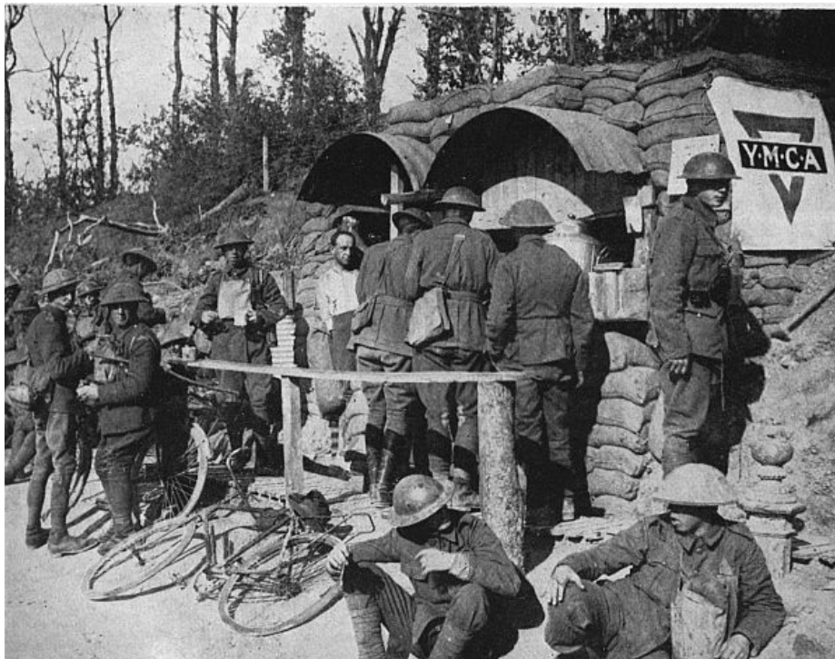
THE RED TRIANGLE IN THE SUPPORT TRENCHES
