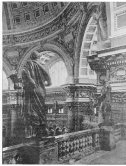
CORNER AT TOP OF STAIRWAY NEW CONGRESSIONAL LIBRARY, WASHINGTON, D.C.
