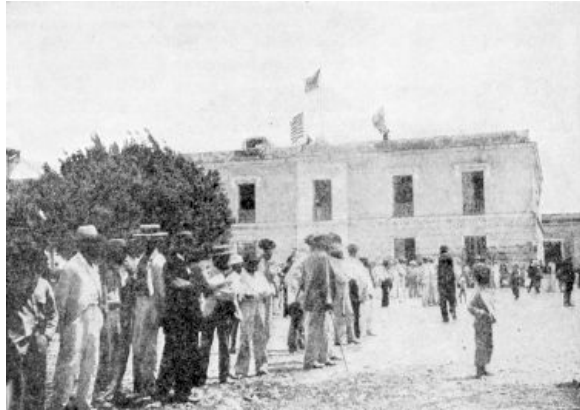
THE CUSTOM HOUSE, PONCE, PORTO RICO, AFTER THE RAISING OF THE AMERICAN FLAG BY GENERAL MILES.
