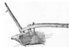
COLONIAL PLOW WITH WOODEN MOULD-BOARD. 1706
