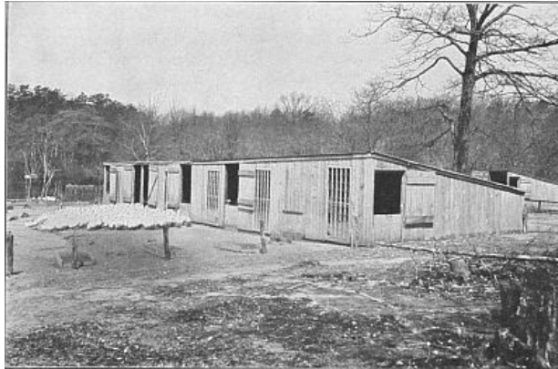
FIG. 18. A good house for breeding ducks. It is 20 feet deep, 40 feet long, 7 feet high in front and 4 feet in the rear and will accommodate 200 breeders. (Photograph from the Bureau of Animal Industry, U. S. Department of Agriculture.)
