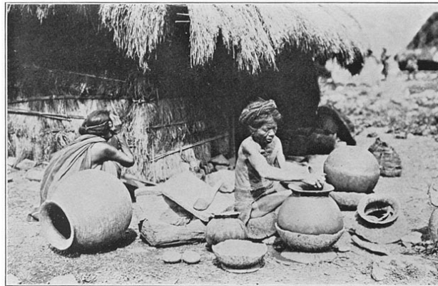
Shaping the rim of a pot
