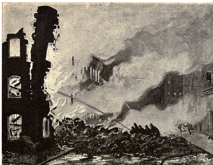
A FALLING WALL.
