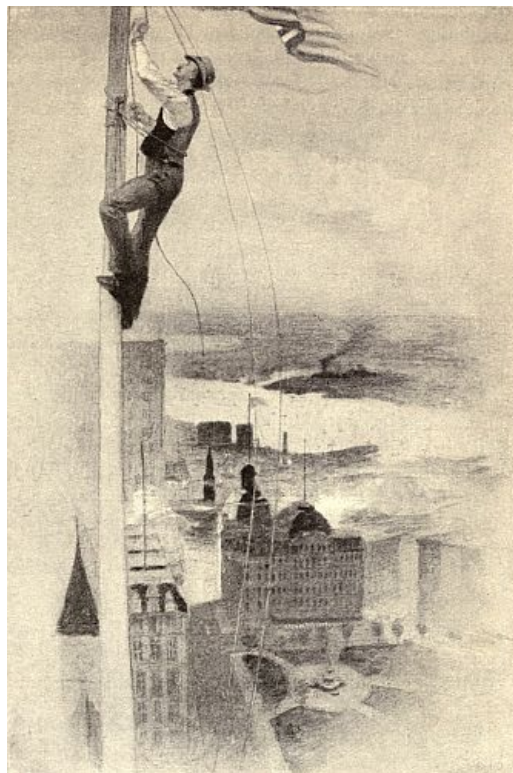
HOW THE STEEPLE-CLIMBER GOES UP A FLAGPOLE.
