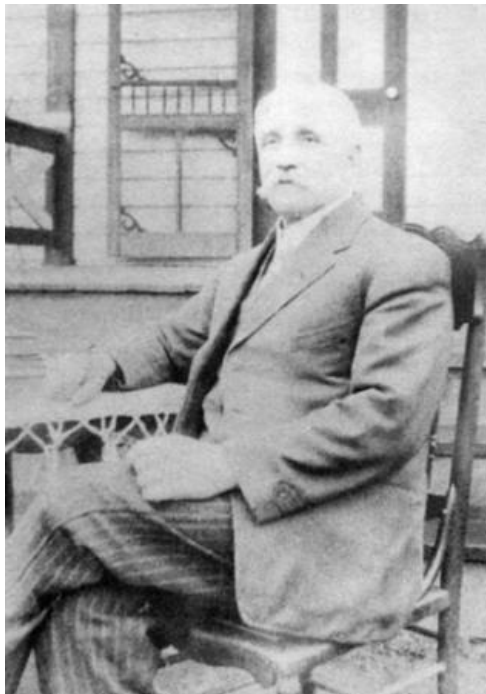
Mr. Jack Walker, the engineer in charge of the construction of the Floris School 1920. Copy of photo in Virginia Collection, Fairfax County Public Library.
