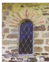
095. Saint-Jean-le-Thomas. The pre-Romanesque choir. The centering of this small pre-Romanesque bay is made with brick quoins. The same bays are present in the church Notre-Dame-sous-Terre, built around the same time in the innards of Mont Saint-Michel. Photo by Claude Rayon. [Claude-30]
