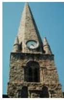
067. Saint-Pair-sur-Mer. The Romanesque tower is square, and its two floors are topped by an octagonal spire. A group of two blind arches adorn the first floor, at the north and south. Large twin bays adorn the second floor on all four sides. Divided by a small column with a square abacus and a square base, these twin bays are topped by a semi-circular arch molded with a simple torus and resting on attached columns. Photo by Alain Dermigny. [Alain-035]
