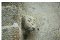
029. Bréville. Above the Romanesque gate in the south base of the tower, a human head carved in a limestone didn't resist well to the test of time, unlike the heads carved in granite in the south gate of the church of Yquelon. Photo by Alain Dermigny. [Alain-013]
