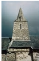
026. Bréville. The first floor and spire of the church tower. The first floor is opened on each side by a long narrow opening. The octagonal stone spire has angles rounded by tori, with a small gable with thin columns in the extension of each opening. Photo by Alain Dermigny. [Alain-011]
