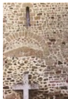
105. Saint-Jean-le-Thomas. The Romanesque murals. The same tympanum of the walled-up gate, seen from the outside. Above the gate, a small Romanesque bay with its centering and abutments in granite. Photo by Claude Rayon. [Claude-29]
