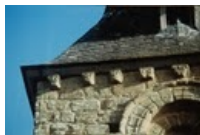
189. Saint-Loup. The Romanesque tower. Detail of the cornice and its modillions carved with human heads. Photo by Alain Dermigny. [Alain-104]
