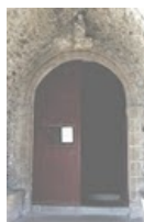
112. Saint-Jean-le-Thomas. The Romanesque gate, in the south wall of the nave. The semi-circular arch of the gate is formed of a grain adorned with a simple torus molding. The arch rests on two attached columns that seem an extension of the torus, with the same diameter. The columns are topped with capitals with a square abacus. The capital baskets are carved with barely visible small angle hooks. The square base is topped by a double torus. Photo by Claude Rayon. [Claude-55]
