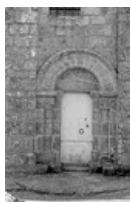
190. Saint-Loup. The Romanesque south gate, in the first row of the choir. The semi-circular arch is formed of an grain surrounded by an archivolt made of a chamfered band. The grain is molded with a thick angle torus followed by a listel and a large shallow cavetto. The grain rests on two attached columns. The capital baskets carved with human heads are topped with abaci molded in quarter-round. Photo by Marie Lebert. [Marie-21]
