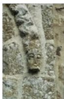
030. Bréville. The Romanesque gate in the south base of the tower. The archivolt topping the semi-circular arch rests on a granite stone carved with a human head. Photo by Alain Dermigny. [Alain-014]
