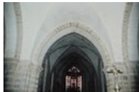
147. Genêts. The Romanesque transept crossing. The piers support four thick slightly triangular arches that surround the groin vault above the transept crossing. Photo by Alain Dermigny. [Alain-079]
