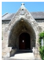
111. Saint-Jean-le-Thomas. The Romanesque gate and its porch, in the south wall of the nave. Like often in the region, a porch was built later on — this one is from the 15th century - to offer to pilgrims and parishioners two stone benches and a shelter from rain and western winds coming from the sea. Photo by Claude Rayon. [Claude-54]
