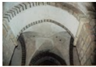
069. Saint-Pair-sur-Mer. The Romanesque tower. Inside, the tower rests on four massive symmetrical piers supporting four slightly triangular arches. These arches surround the groin vault beneath the tower. Photo by Alain Dermigny. [Alain-036]
