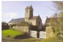
082. Angey. The church, with its Romanesque choir. The base of the tower may also be Romanesque, but from a later period, because its masonry is slightly different from the masonry of the choir. Photo by Claude Rayon. [Claude-25]
