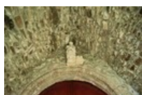
114. Saint-Jean-le-Thomas. The porch. The stone roof of this 15th century porch is made of irregular schiste plates joined with a thick mortar. The arch of the Romanesque portal is adorned with a torus. Photo by Alain Dermigny. [Alain-060]
