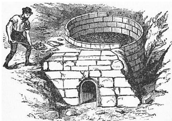
FIG. 4.—Roman kiln found at Castor. The low arch is for the insertion of the fuel; the pots rested on the perforated floor, made of clay slabs; the top of the kiln is missing,—it was probably a dome.
