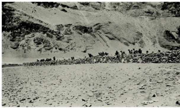
PIONEERS DESTROYING KANGMA WALL.
