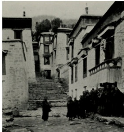
CORNER OF COURTYARD OF ASTROLOGER'S TEMPLE, NECHANG.
