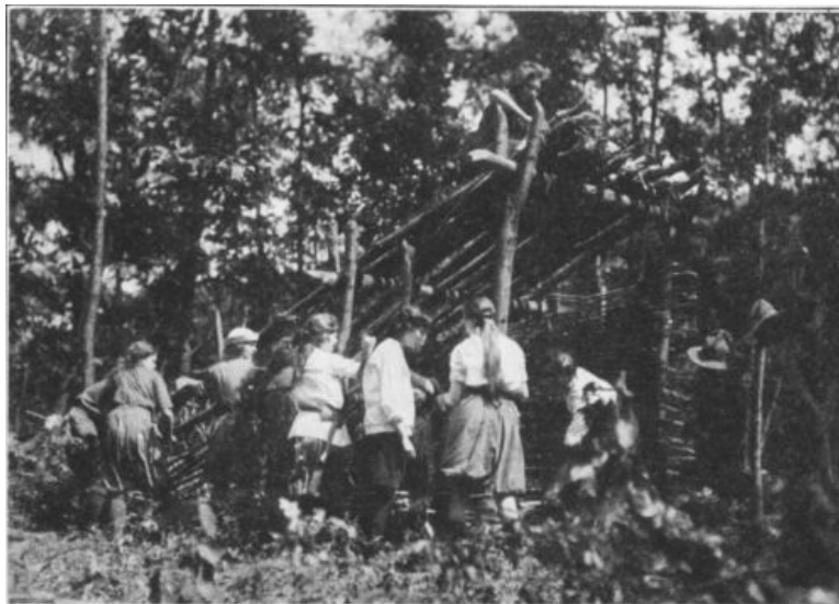
THE LEAN-TO GOING UP
