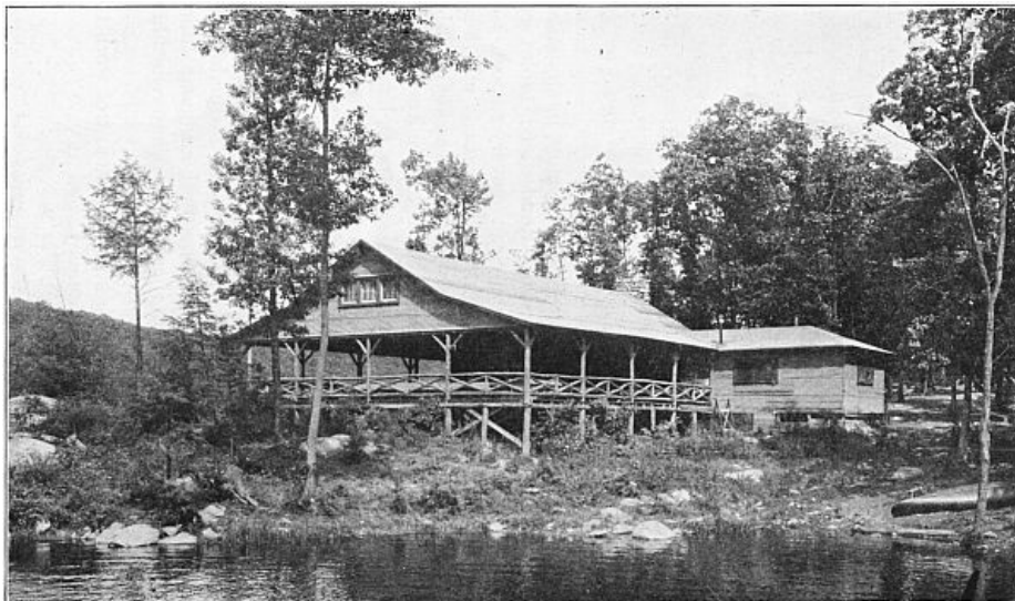
This Mess Hall is open to wind and sun, but rolled up canvas walls are ready to be dropped.
