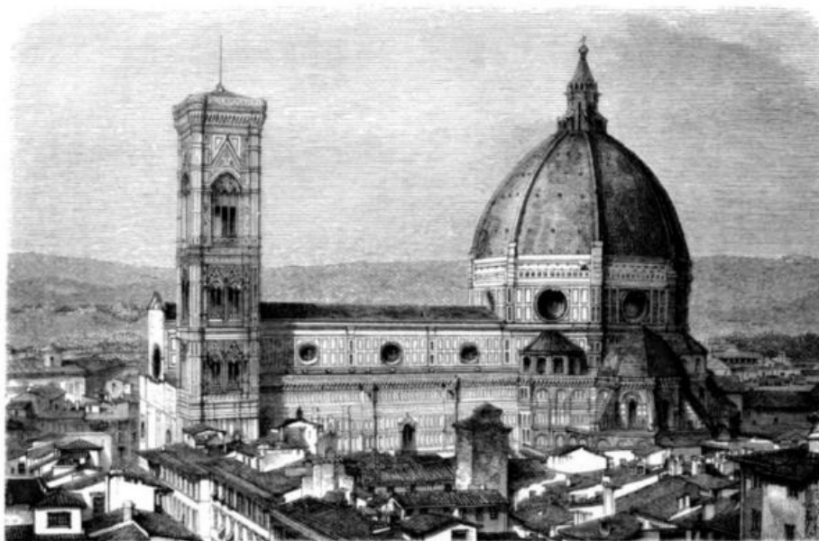
FIG. 51.—THE CATHEDRAL AT FLORENCE. WITH GIOTTO'S CAMPANILE. (BEGUN, 1298; DOME, 1420-1444; CAMPANILE BEGUN, 1324.)
