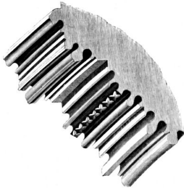
FIG. z.—ARCH MOULDING. (Gothic, 13th Century.)
