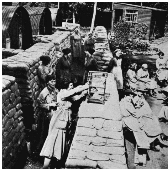
WAAC ENCAMPMENT PROTECTED BY SANDBAGS
