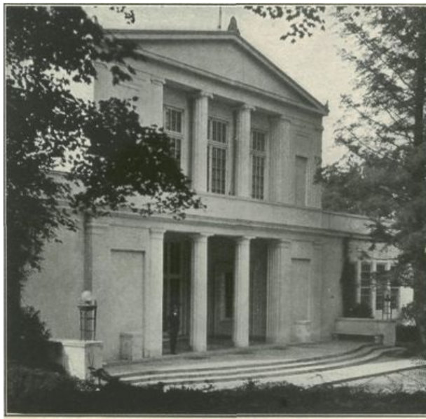
Exterior of the Beechwood Theatre.
