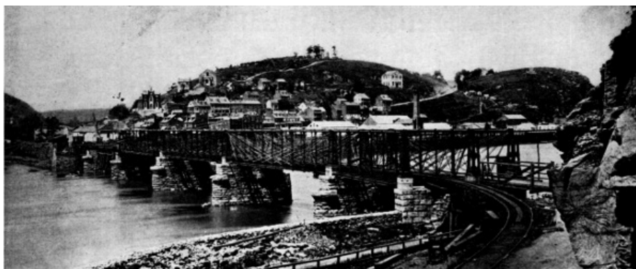
Figure 13.—THE FOUR BOLLMAN SPANS at Harpers Ferry that survived the Civil War. The spans were completed in 1862-1863. (Photo
