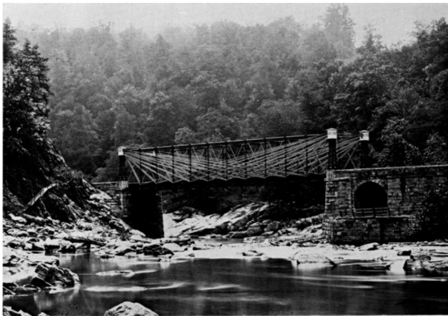
Figure 19.—PATAPSCO RIVER CROSSING of the Baltimore and Ohio between Thistle and Ilchester, Maryland. (Photo 695, Baltimore and Ohio Collection, Museum of History and Technology.)
