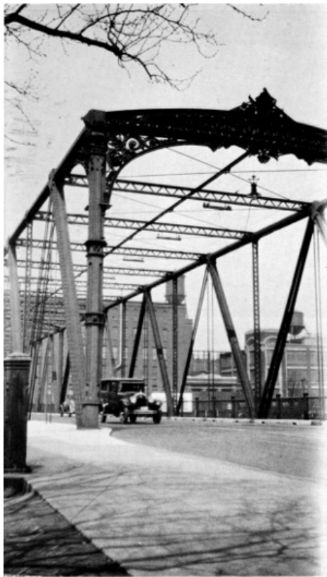
Figure 15.—NORTH STREET (now Guilford Avenue) bridge, Baltimore. In this transitional composite structure cast iron was used only in the relatively short sections of the upper chord. For the long unsupported compression members of the web system, standard wrought-iron angles and channels were built up into a large section. The decorative cast-iron end posts were non-structural. (Photo in the L. N. Edwards Collection, Museum of History and Technology.)
