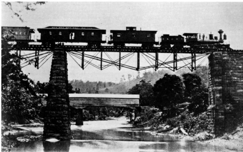
Figure 10.—POTOMAC RIVER CROSSING of the Baltimore and Ohio at North Branch, Maryland, built in 1856. There are three Bollman deck trusses. (Photo courtesy of Baltimore and Ohio Railroad.)
