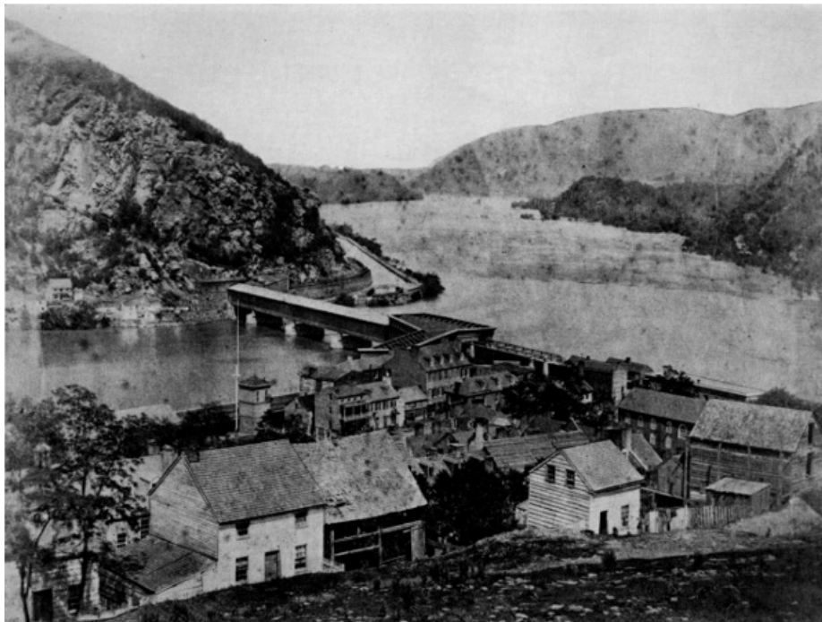
Figure 8.—THE BALTIMORE AND OHIO RAILROAD'S Potomac River crossing at Harpers Ferry, about 1860. Bollman's iron "Winchester span" of 1851 is seen at the right end of Latrobe's timber structure of 1836, which forms the body of the bridge. (Photo courtesy of Harpers Ferry National Historical Park.)
