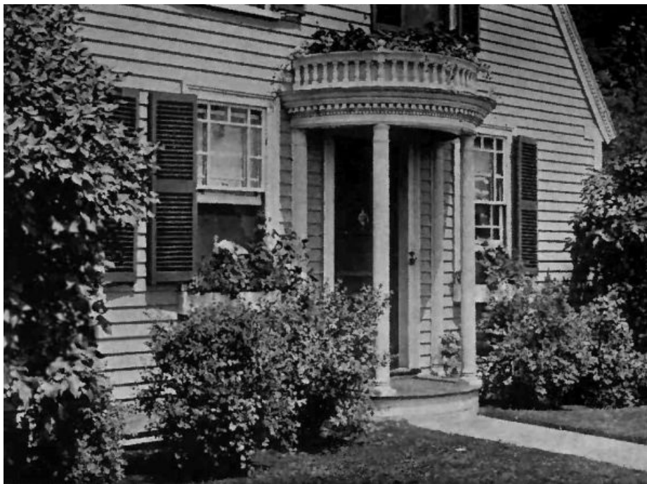
The Entrance Porch
