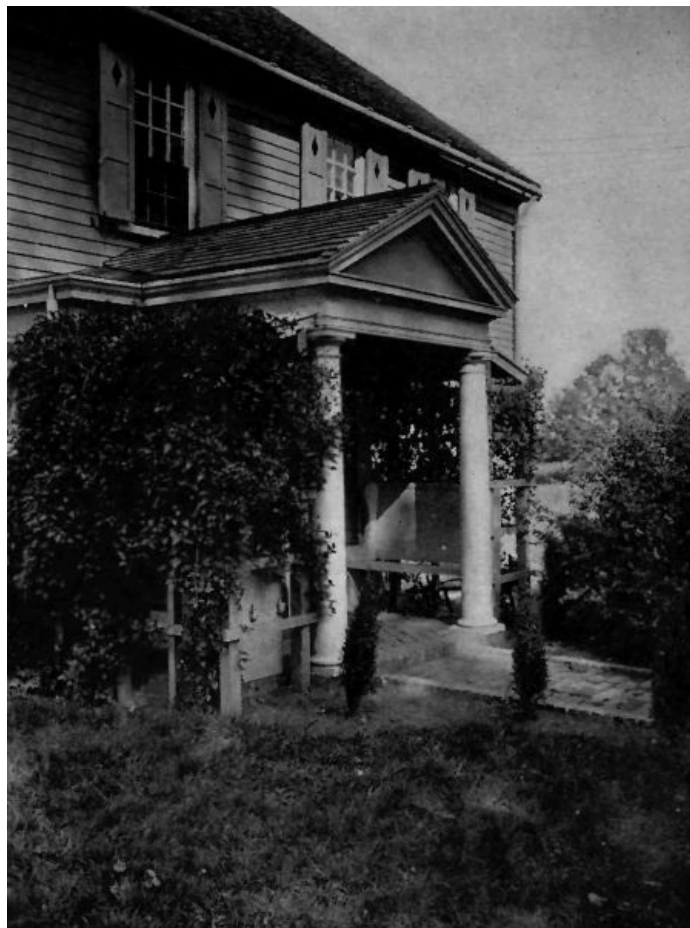
The Entrance Porch
