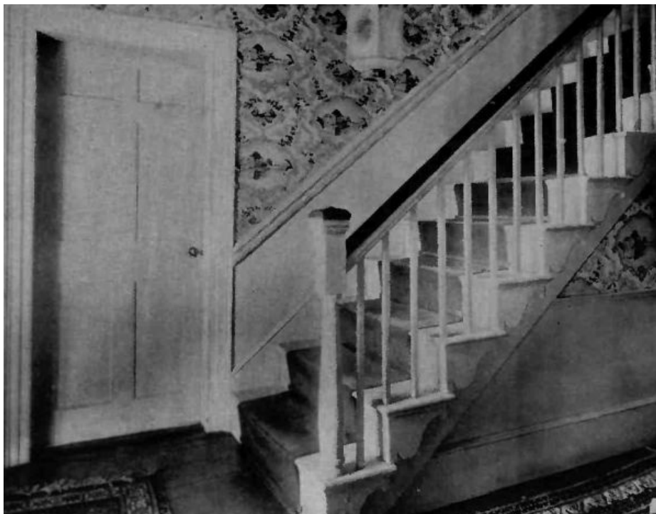
The Hall and Stairway
