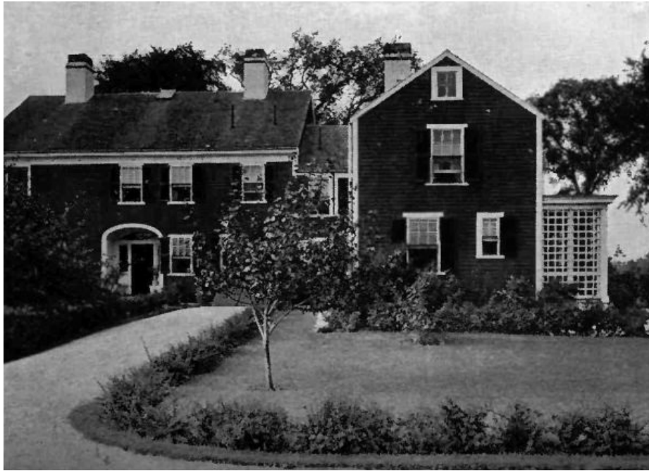
The Service Wing
